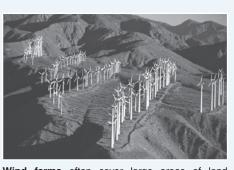
Wind farms often cover large areas of land but turbines can be designed to operate at sea and, on a smaller scale, along highway edges. Turbines range in size from just a meter across, to the world's current largest at 198 m tall and 126 m in diameter, with a generation capacity of 7 MW. Larger 10 MW turbines are already being planned.
