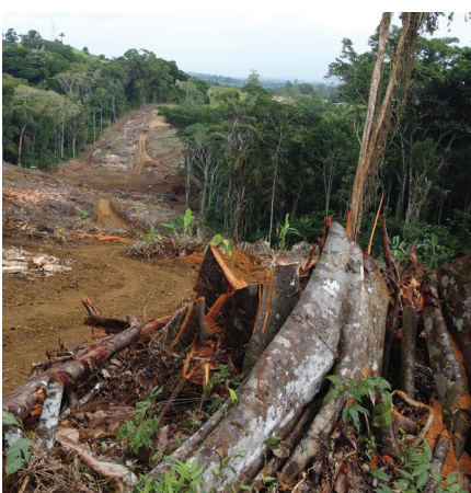
New road to Ilhéus, Bahia, Brazil: The building of new road networks into regions within tropical rainforests causes considerable environmental damage. In areas with very high rainfall there is an increased risk of erosion and loss of topsoil.
